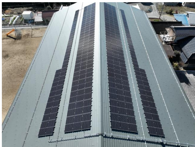
REC製：REC365TP4M 365W×156枚
