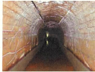
[幹線水路]隧道:補修(無機系被覆・裏込注入)
