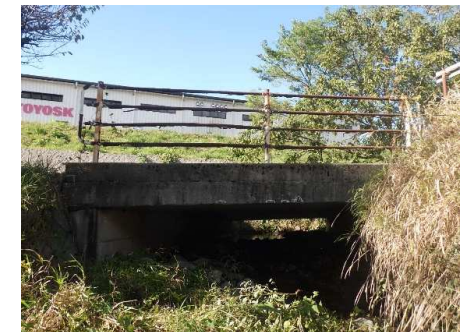
③ RC床版橋 L=5.5m
