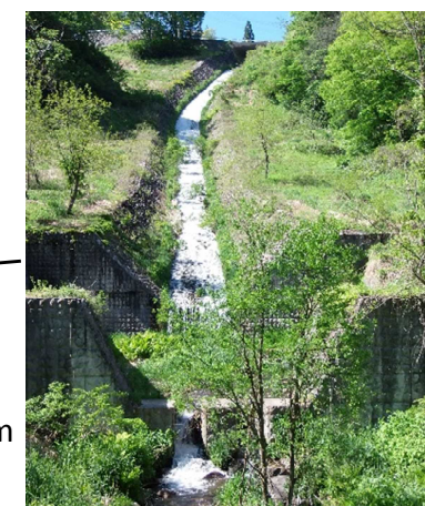
カクレ沢 鋼製枠堰堤 H=8m,L=137m,V=5,700m 3
